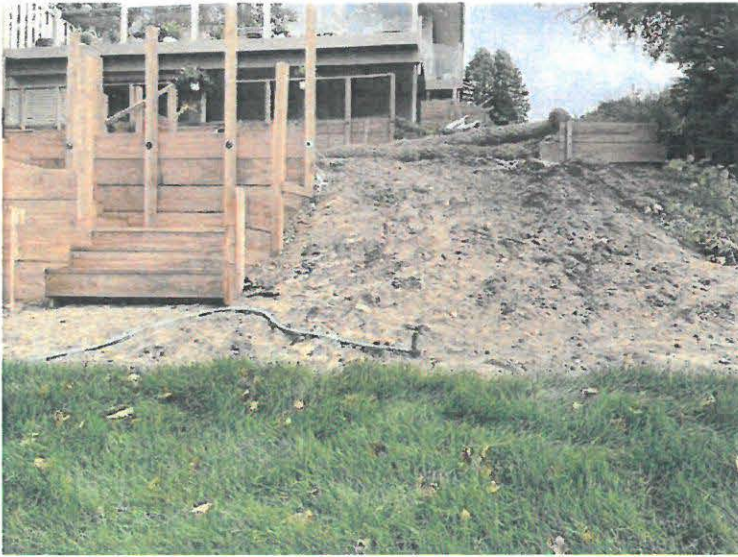
Photo 5 – Looking east from existing retaining wall up the south property line at the new intermediate timber retaining wall and stairs. This unrestored area is the location where up to 4' of fill is proposed.
