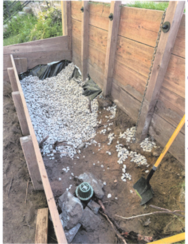
12) Outlet Fix. 70% Drain Stone
