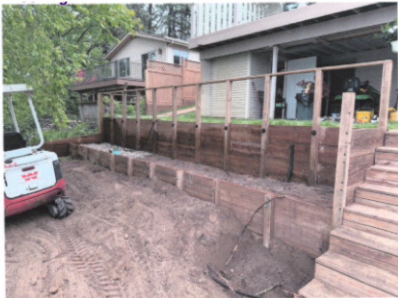
15 & 16) Outlet Fix Terrace Extension 90% backfill, Looking NE.
