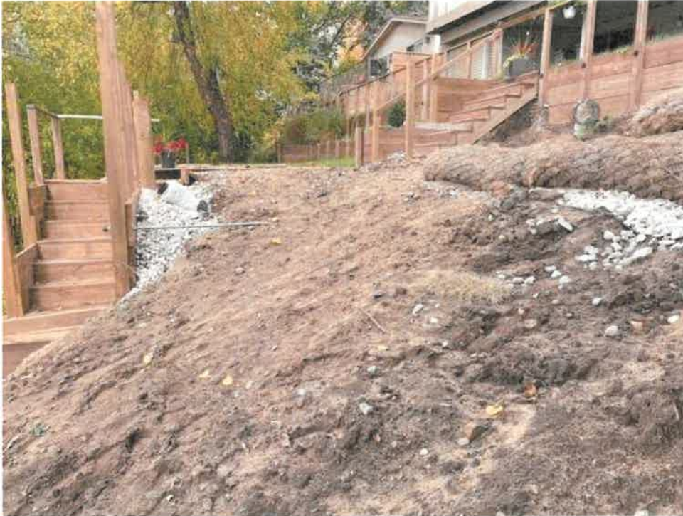
Photo 1 – Looking north from south property line detailing French drain outlet into stone fill of lower retaining wall.
