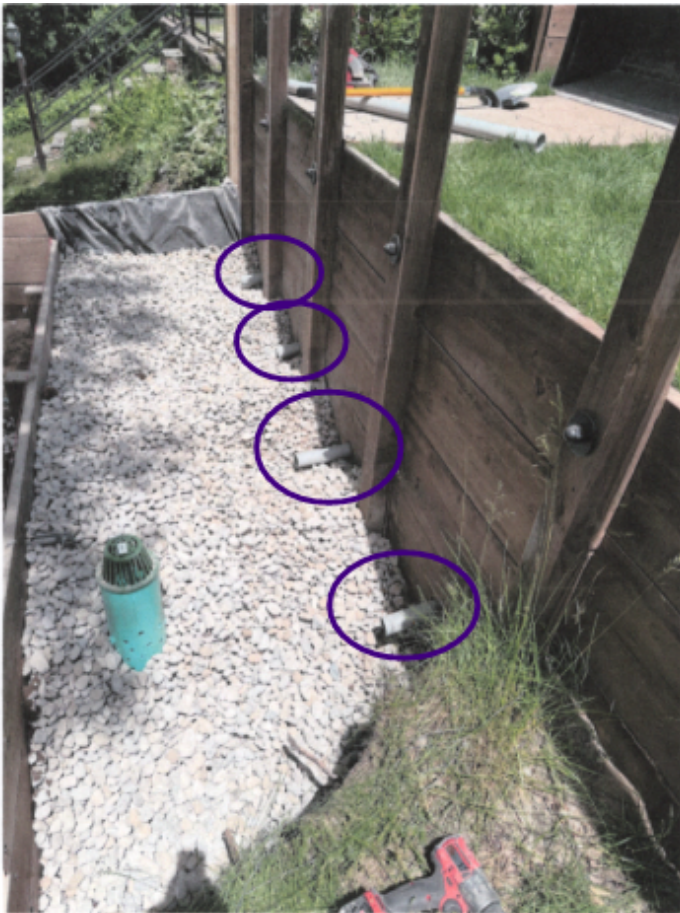
11) Outlet Fix 50% Drain stone, Note Weep Hole Pipes .
