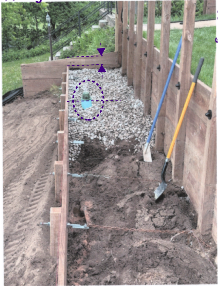
14) Outlet Fix Terrace Extension 90% backfill, Note Riser for Overflow set below wing wall. Looking N.
