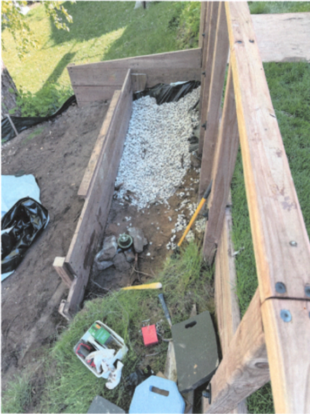
11) Outlet Fix 50% Drain stone, Note Weep Hole Pipes .
