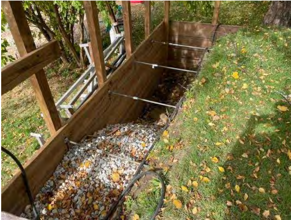
Photo 7 – Detail of clean stone infill between new and existing lower retaining wall.
