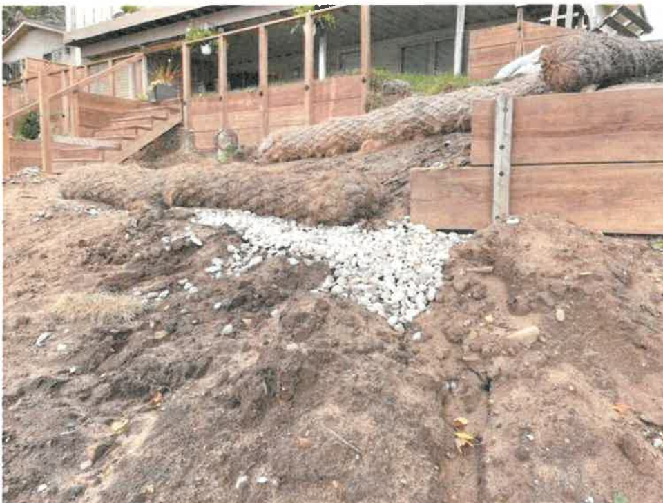
Photo 1 – Looking north from south property line detailing French drain outlet into stone fill of lower retaining wall.
