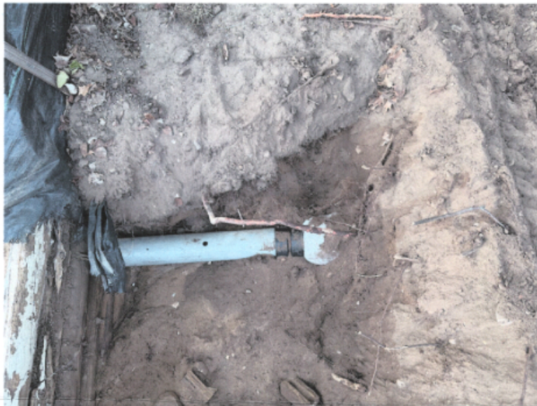
7) Overflow connected to outlet pipe
